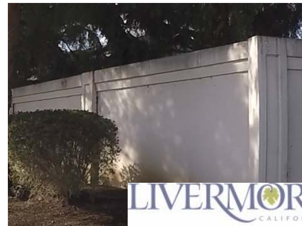
Concrete Pre-cast Panels
